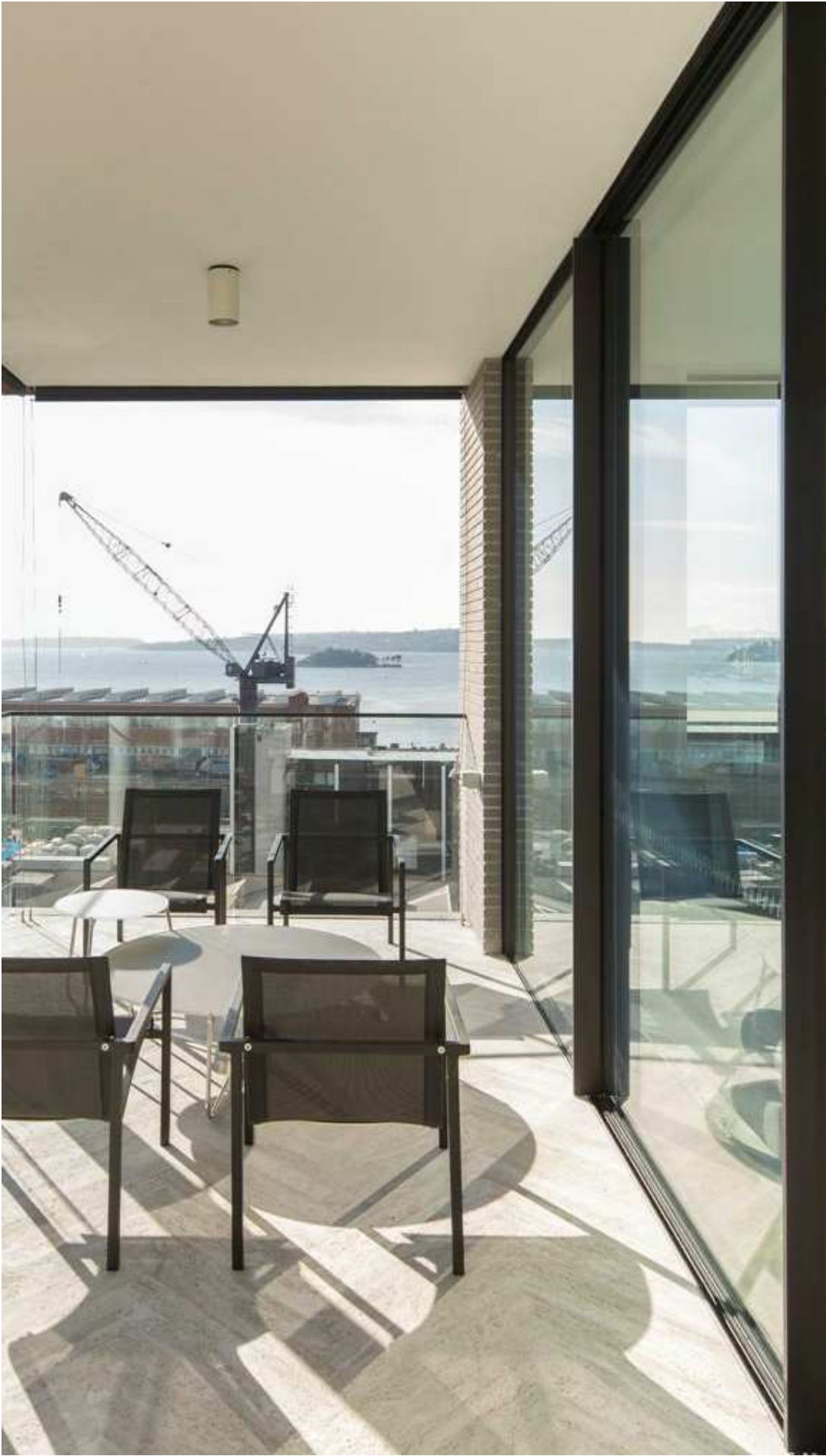
Aluminium framed windows Material:Aluminium Finish/ Colour: Powdercoat, Dark Grey
