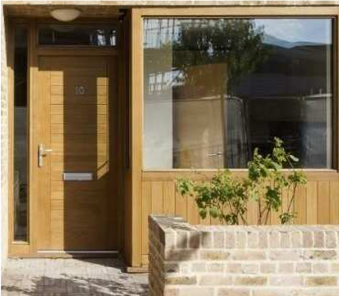
Timber framed windows Material:WRC or similar Finish/ Colour: Clear Oil
