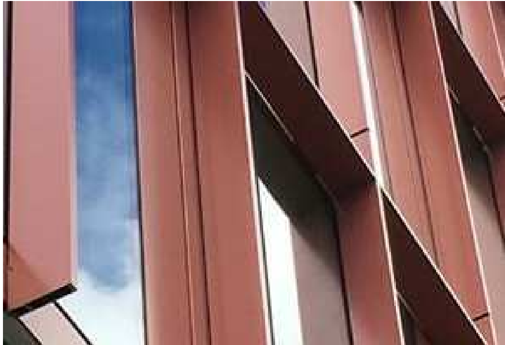
Aluminium Window Fin Material:Aluminium Finish/ Colour: Powdercoat, Pink/ red tone from brickwork
