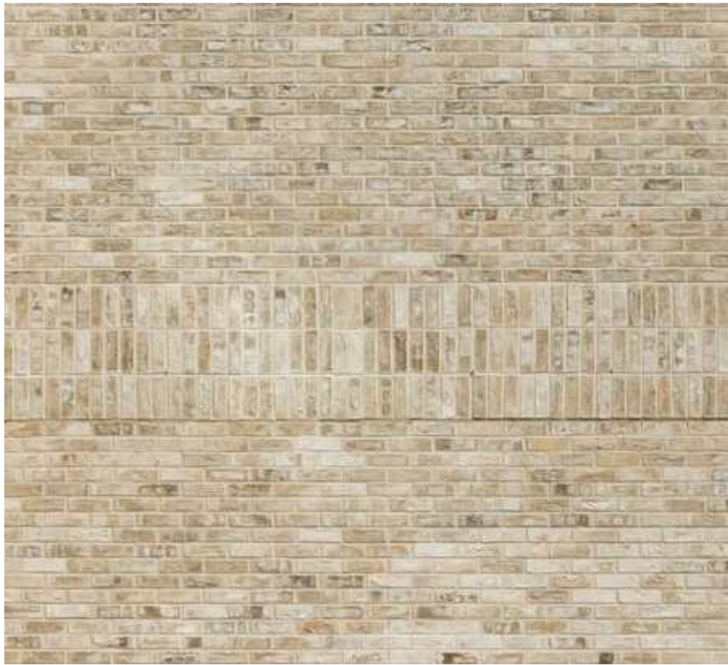
Face Brickwork Detail Spandrel Panel and Ground Floor Brick Soldier Course
